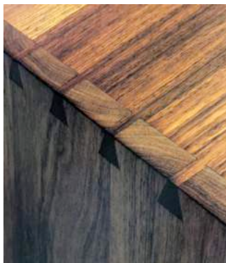
Figure 17: Dovetail Joints (George, 1981)
